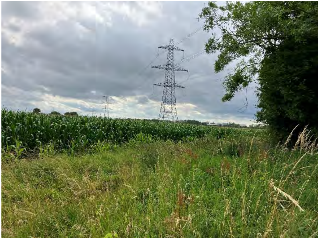
Plate 1: View of project substation and POC area from the north-eastern end, facing south-west
